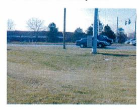
This small detention basin will be affected by Alternate 2 or 3. It will be difficult to maintain the existing basin volume with surface detention. Underground detention would be a good application with this situation in the event that Alternate 2 or 3 is constructed.
