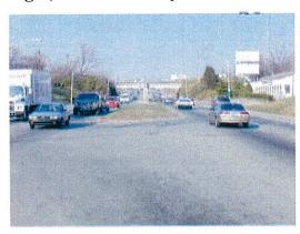
Flooding is also known to occur in this location along New Circle Road beneath the CSX railroad bridge. The storm water piping system is inadequate to handle heavy rainfall amounts.
